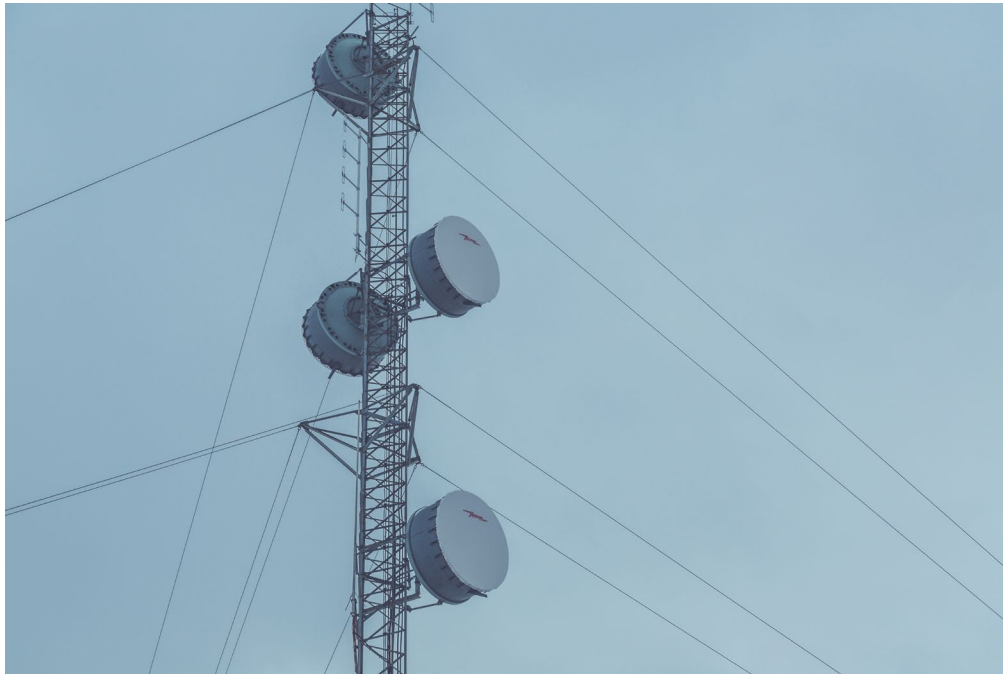
Point-to-point microwave links use highly directional antennas
