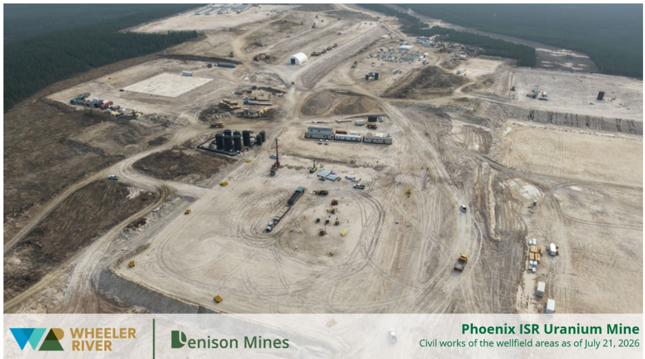
Figure 2. Phoenix ISR Mine, Civil Works for Wellfield, Process Plant, and Substation Areas as of July 21, 2026
