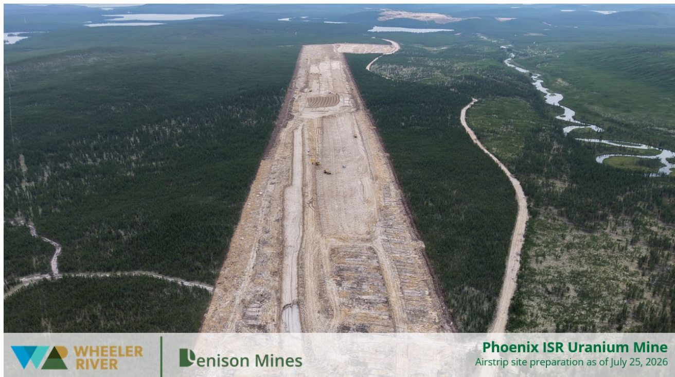
Figure 4. Airstrip Site Preparation (Phoenix site in the distances) as of July 25, 2026
