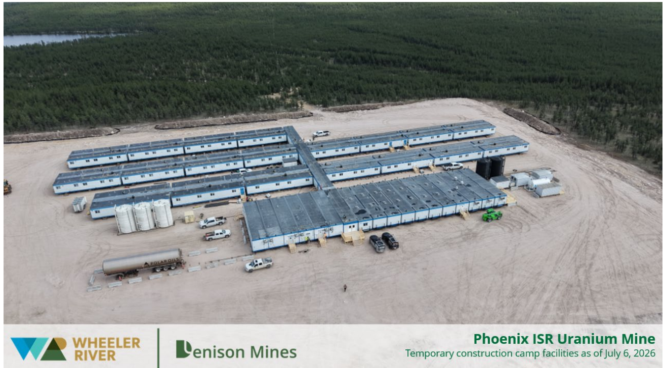
Figure 3. Temporary Construction Camp Facilities Installation Progress at the Phoenix Site as of July 6, 2026
